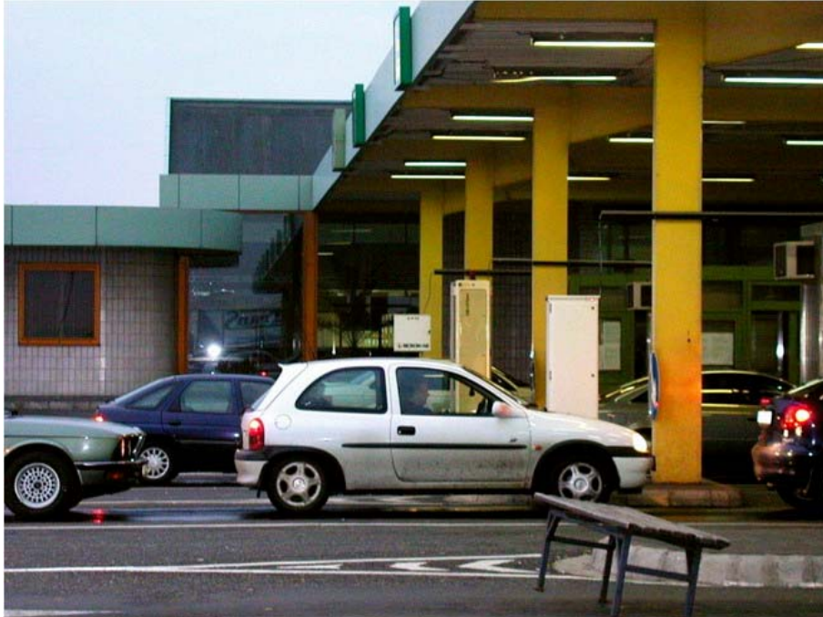
Figure 2 - Portal monitors to detect radioactive sources in road transport at border crossings
